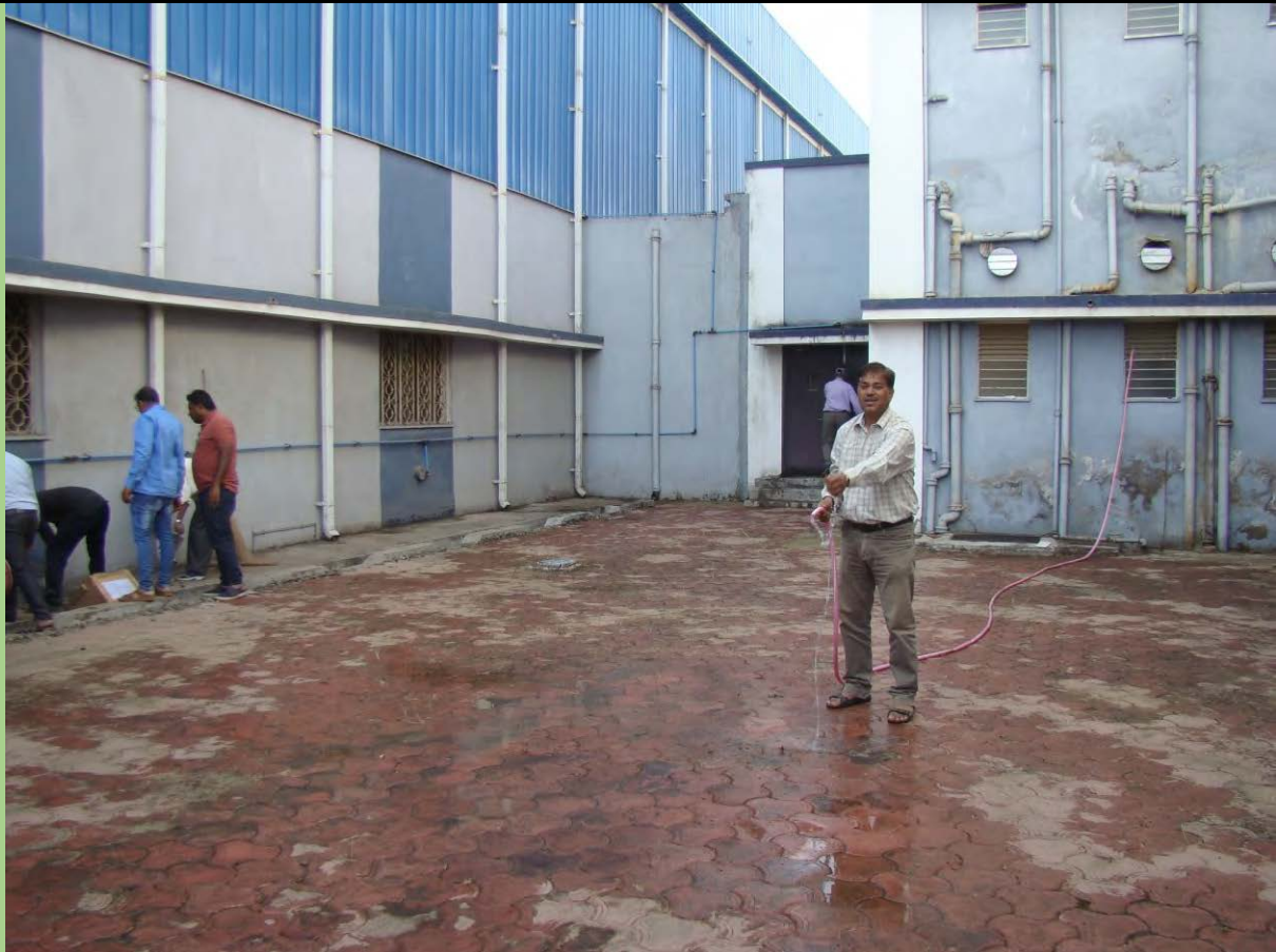
Final cleaning and washing of cleaned area
