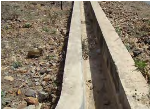
Before cleaning – Trench line
