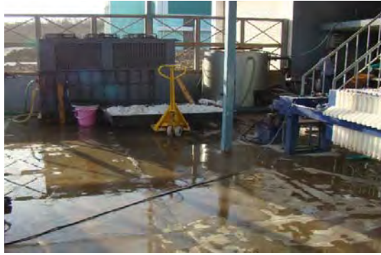
After cleaning – Effluent Treatment Plant area
