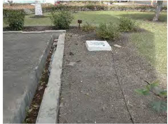
After cleaning near front wall of Block G
