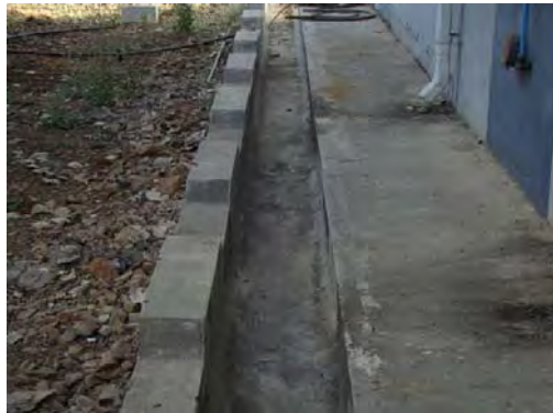
After cleaning – Trench line
