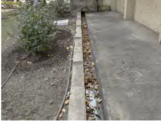
Before cleaning near front wall of back door of Block
