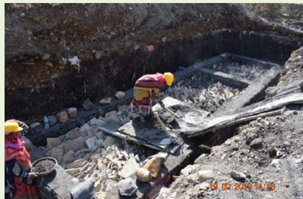
Fig. 33 Reuse of construction debris: Retaining wall for the FEL laboratory extension (2/2).
