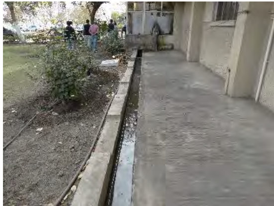
After cleaning near front wall of back door of Block G
