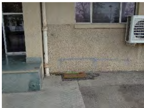
Before cleaning outside front door of Block G
